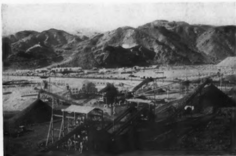
KAISER'S Fontana mill is one of the pioneers in the development of the sintering plant for faster and more economical iron ore beneficiating.
